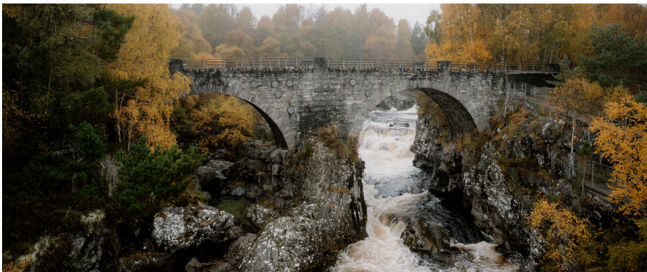
Silverbridge, its two arches over the Black Water Falls
